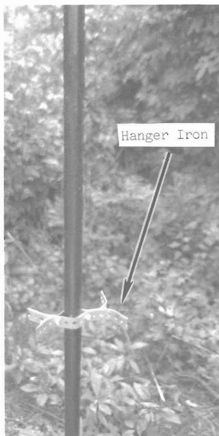
Figure 2. Hanger Iron.
